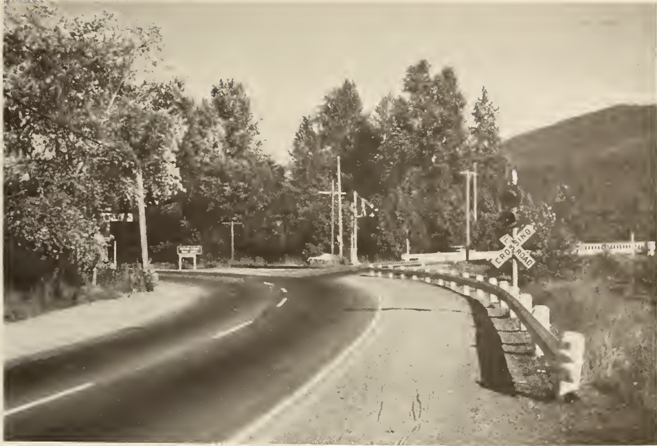
Figure 5 Washington State Installation
